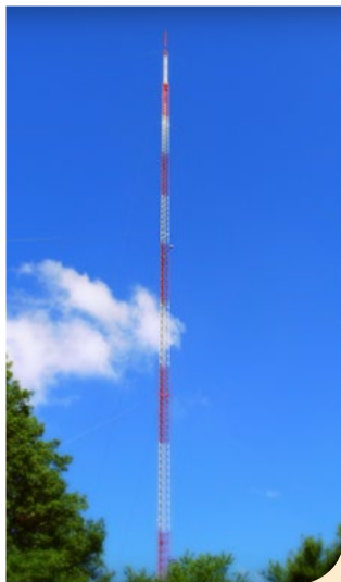
Guy tower constructed by Mercury Communications, Inc.
